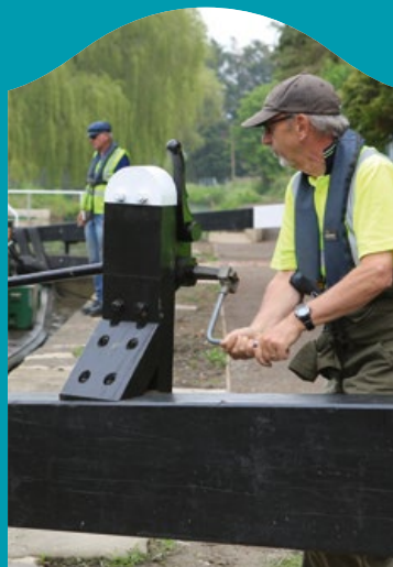
Above: Paddle gear in action
