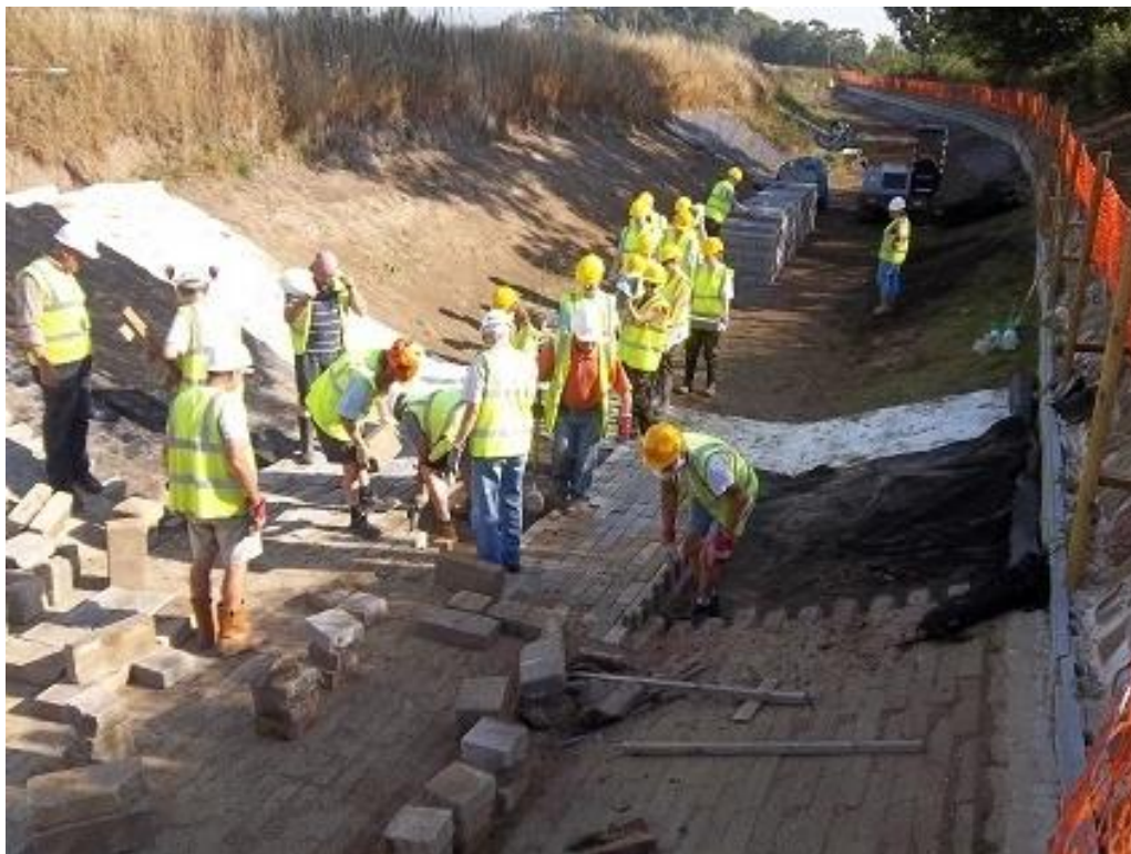
Sahara acrylic lining system: Montgomery Canal, Redwith Bridge to Pryces Bridge
