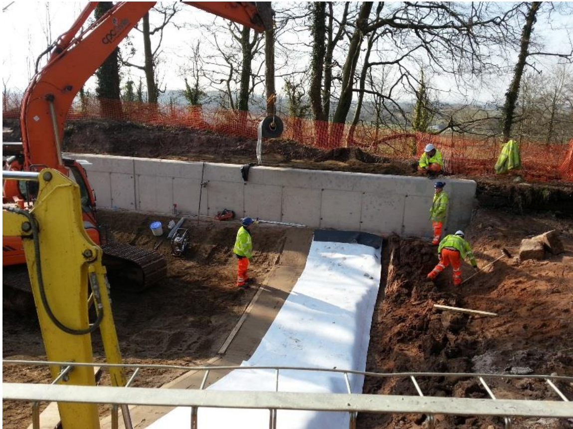
Sahara acrylic lining system: Montgomery Canal, Redwith Bridge to Pryces Bridge
