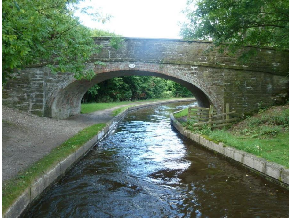
Reinforced concrete channel lining system: Llangollen Canal, near Llangollen
