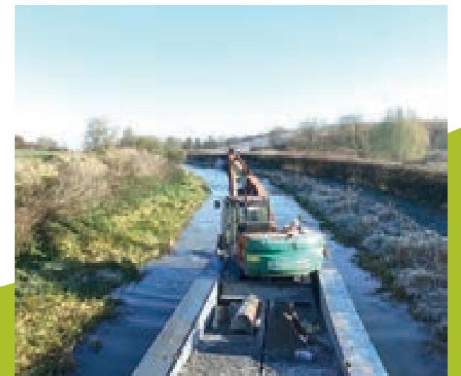
Dredging to remove sediment from the channel
