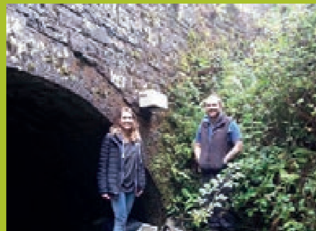
Volunteers installing a dipper box on an aqueduct on the Monmouthshire and Brecon Canal
