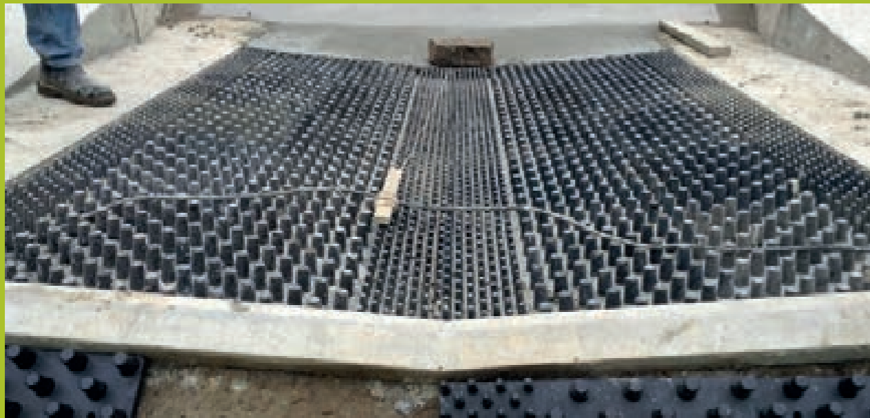
Newly installed eel tiles on a weir. Once completed, water will run down these tiles so that eels can wriggle their way up © Environment Agency
