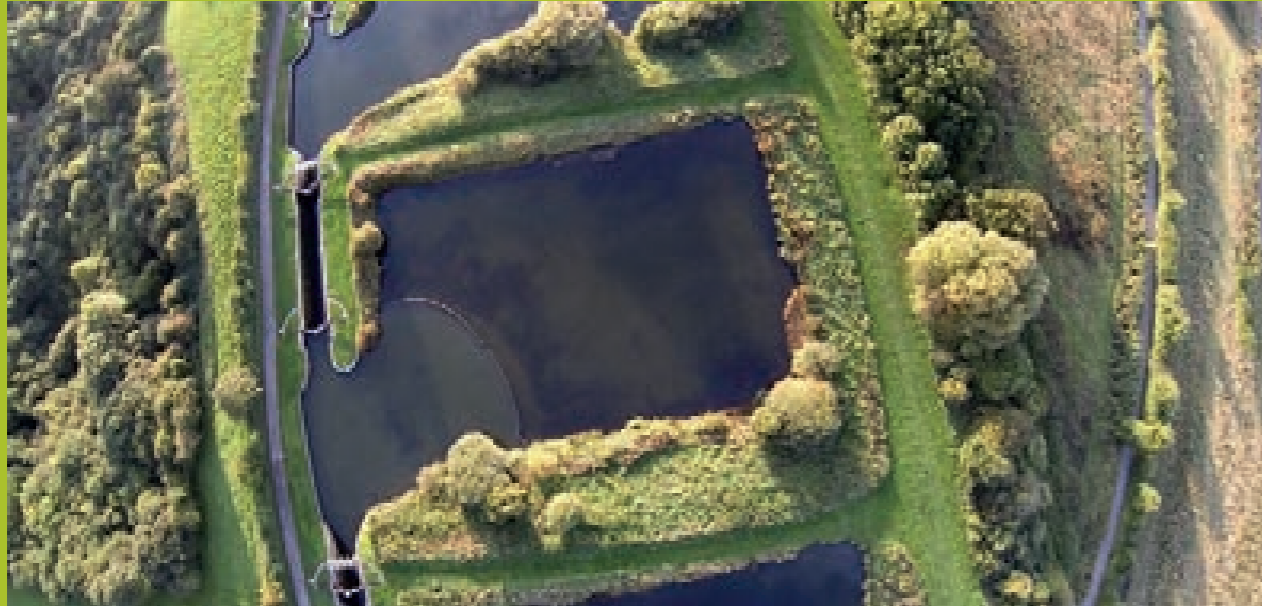
Aerial view showing a silt curtain. You can see the difference in the water quality either side of the curtain. The dark areas are clear water. The brown water contains much more suspended sediment
