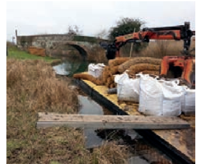
Coir rolls ready for installation, used to rebuild reed fringes. These provide habitat for fish and therefore otters
