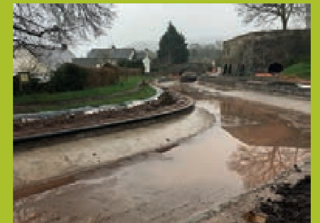
Canal relining underway on the Monmouthshire and Brecon Canal
