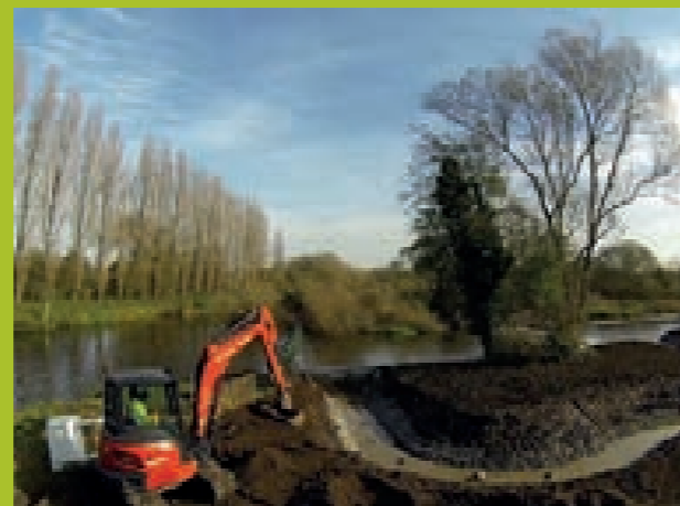
Digging the fish bypass
