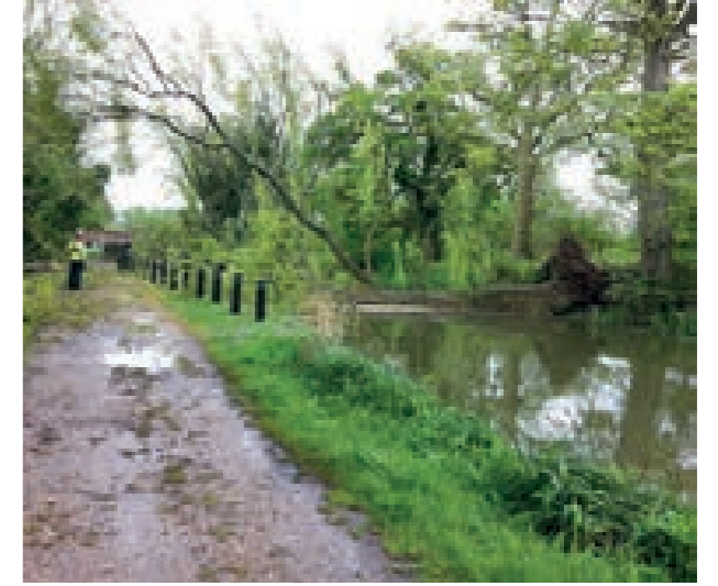
Tree fallen across the channel blocking the navigation, in need of removal
