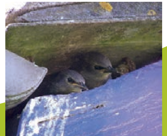
Eaves and roof voids can make good nesting places
