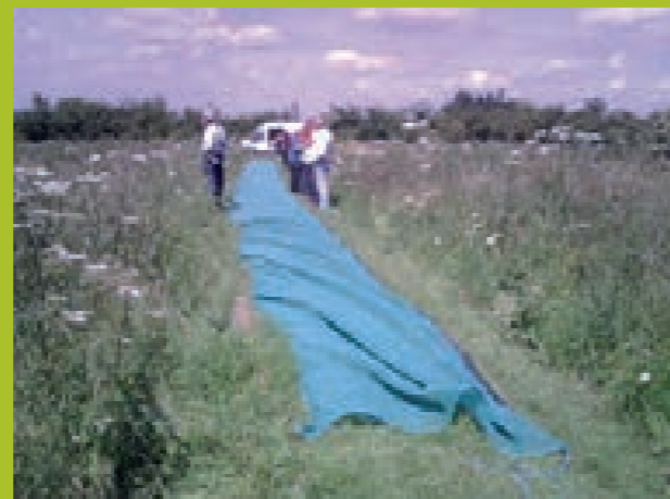
Silt curtain rolled out, ready for installation
