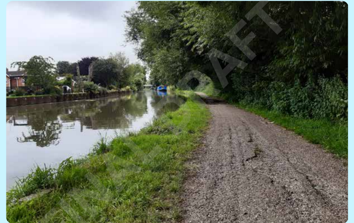
Before and after photos of the towpath improvement works:
