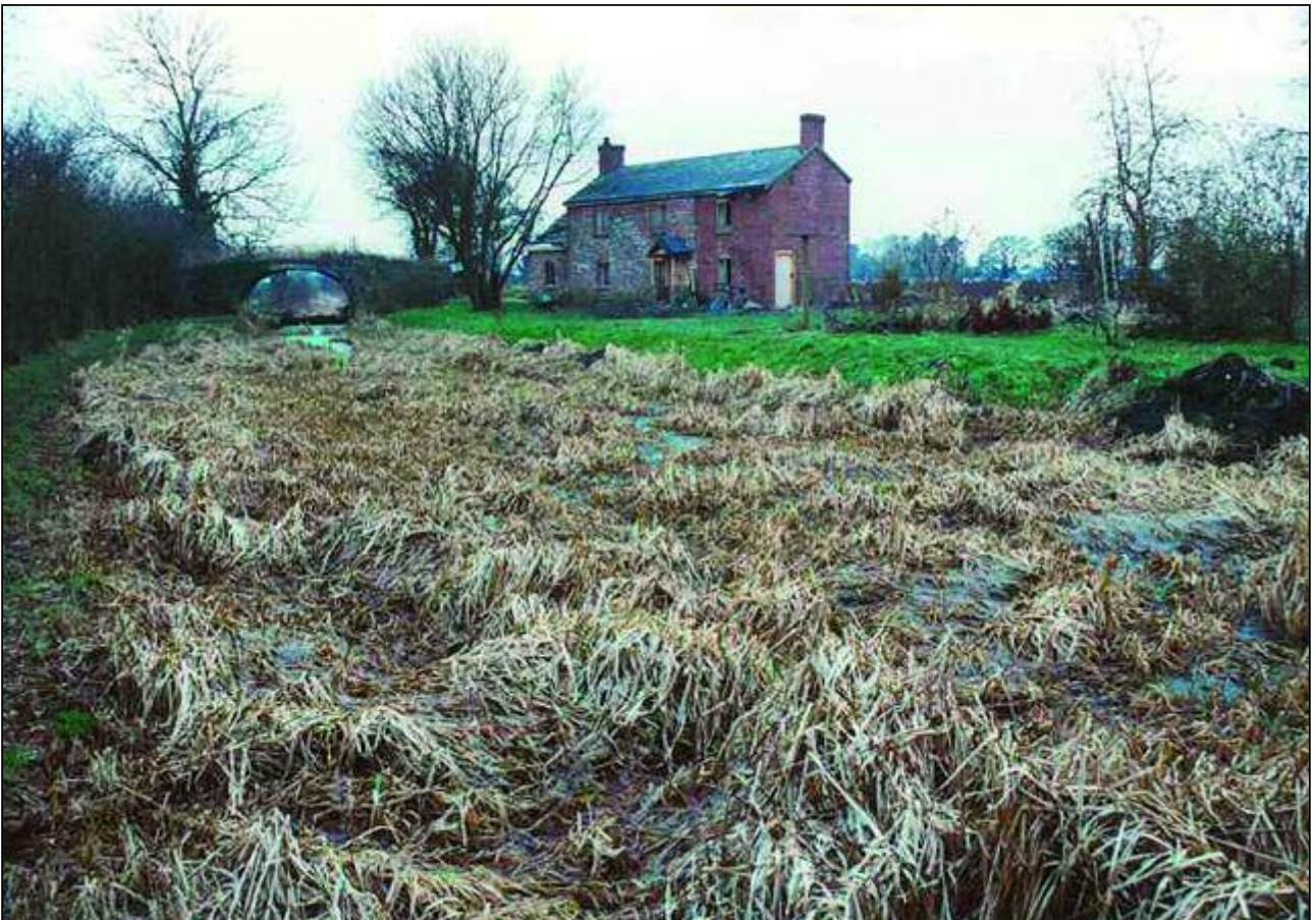
Figure 3.10. Vulnerability: loss of open water on neglected length. Gronwen Wharf, 2000.
