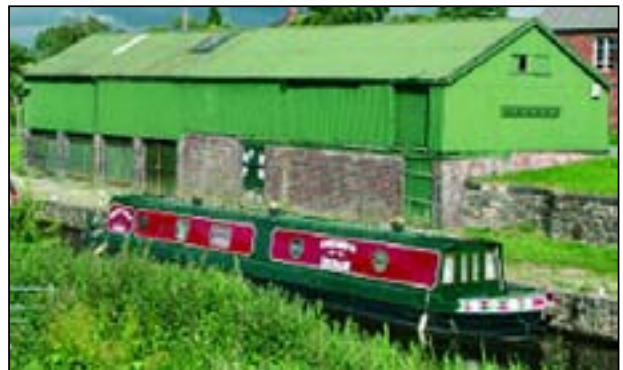
Queen's Head Warehouse.
