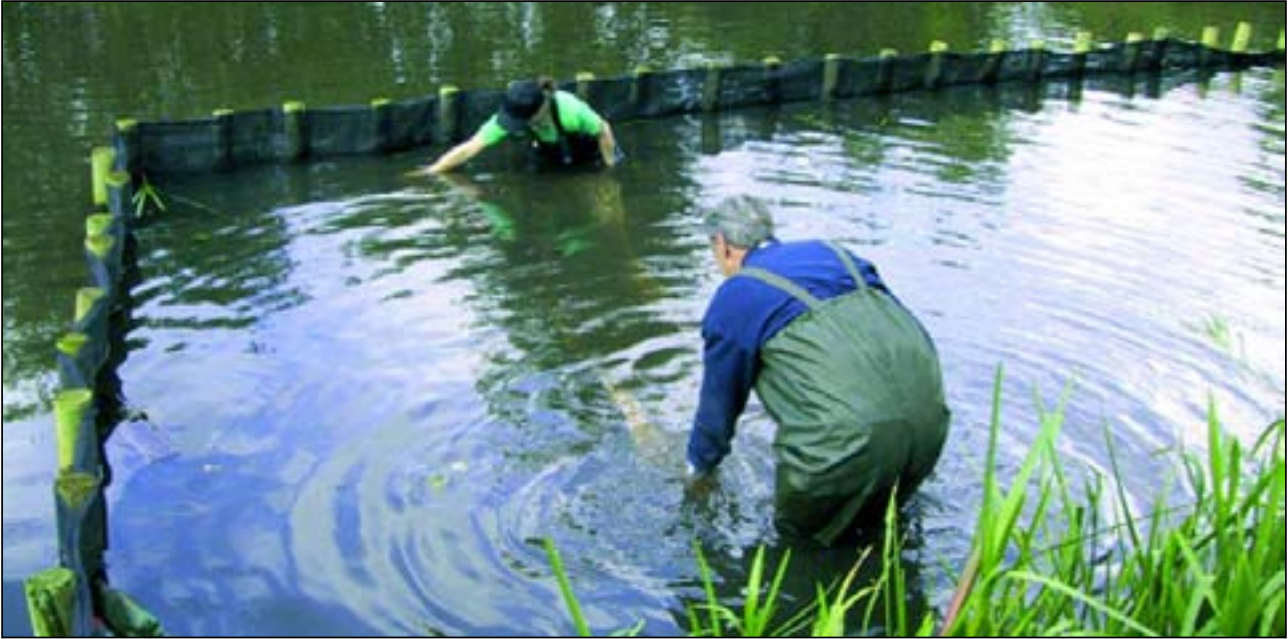
Figure 7.8. On-line conservation, Rochdale Canal, with silt screen protection.
